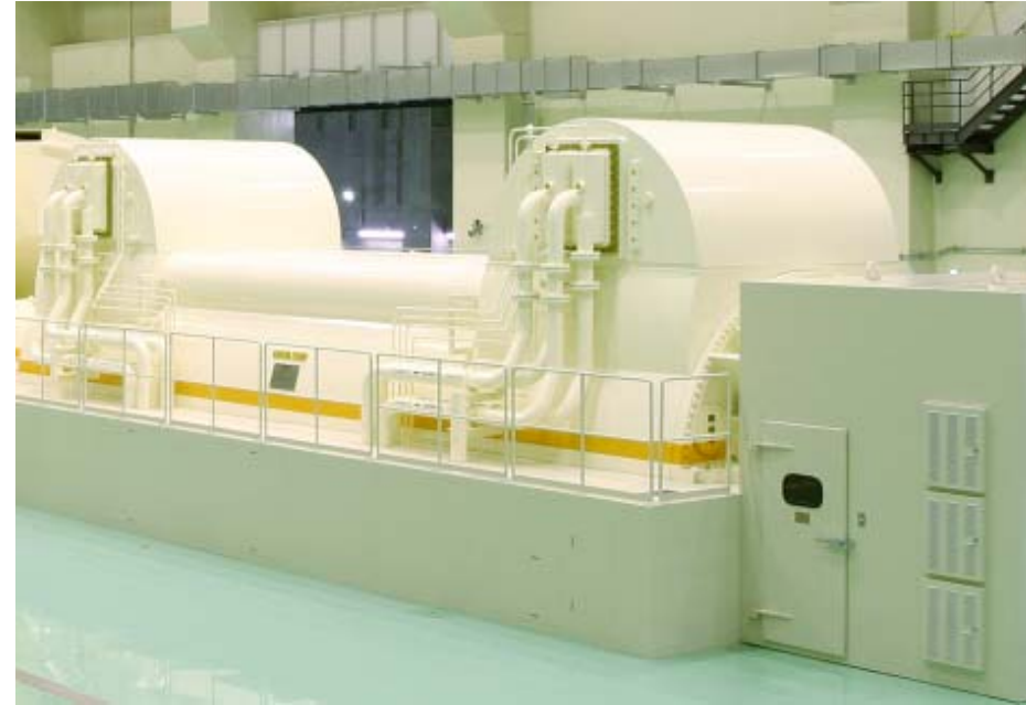
1,570-MVA (1,800 rpm) Turbine Generator at Hamaoka Nuclear Power Station No. 5 (Japan)
